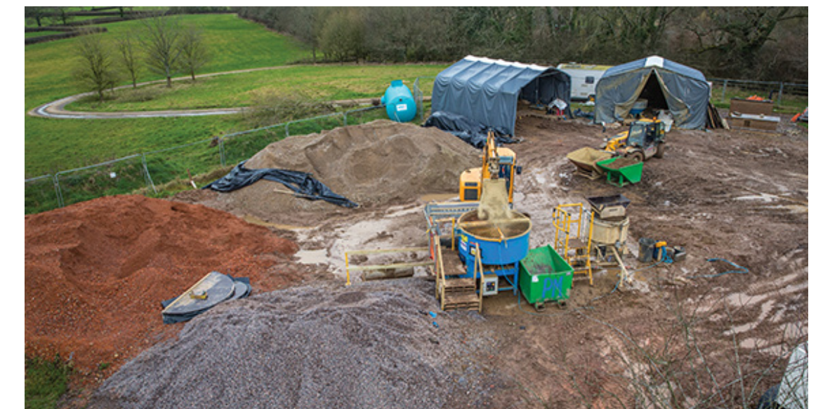
Rammed Earth House Site, Tuckey Design Studio. Image by Jim Stephenson.
